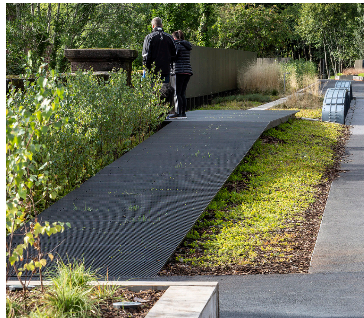
Metal, concrete and stone tie to Waterton Canyon Diversion Dam
