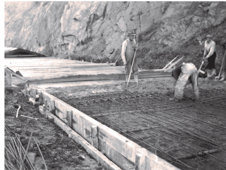
Exhibit 3-6: The bench flume at Waterton Canyon was subject to constant repair. This Nov. 18, 1934, photograph depicts the replacement of the timber floor with a new concrete floor slab. Source: Denver Water, Album 41, page 20, photo #3973.
