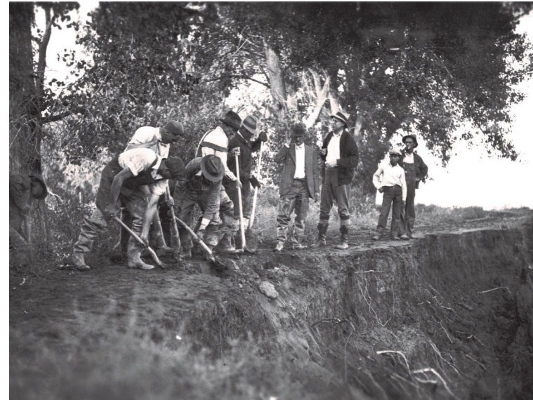
Exhibit 3-5: 1933 repairs to Canal bank washed out by "overtopping during storm." Source: Denver Water, Album 41, page 81, photo #3656.
