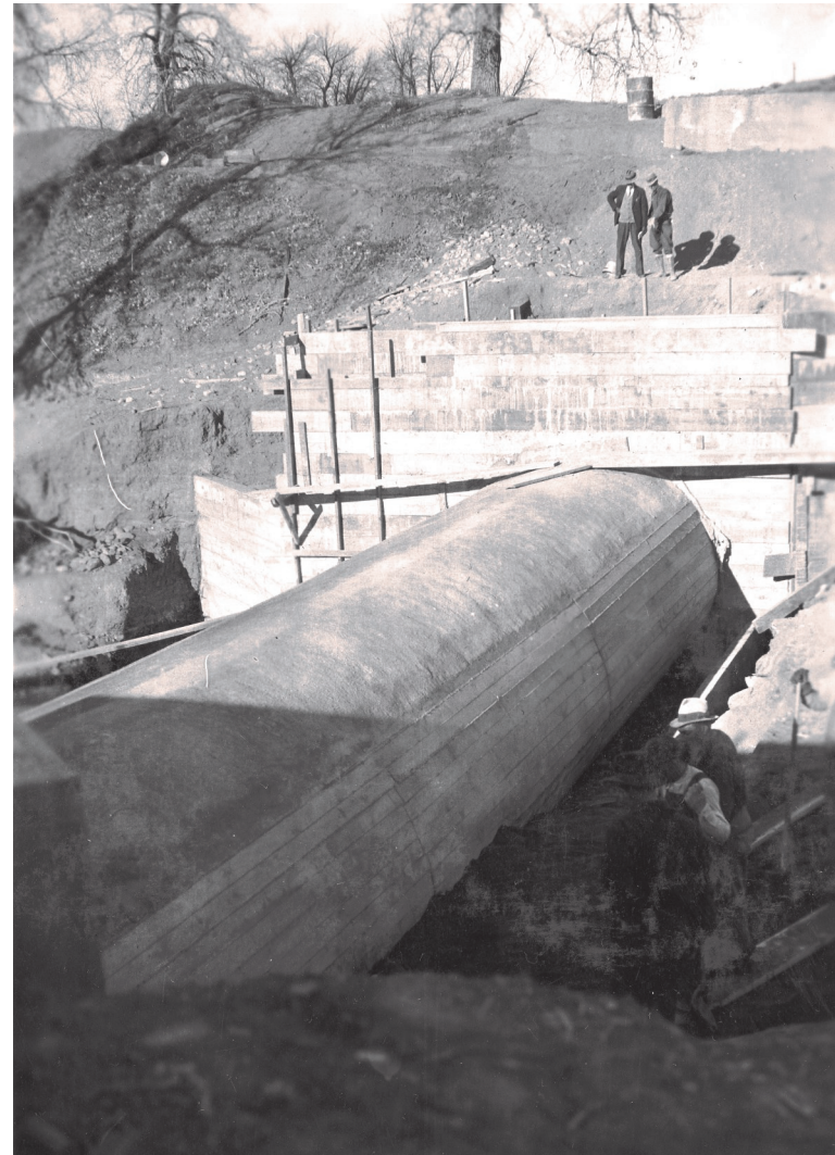
Exhibit 3-8: In February 1934, Denver Water installed a concrete siphon at Little Dry Creek. Source: Denver Water, Album 41, page 30, photo #3790.
