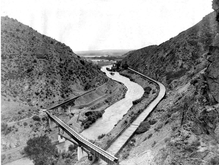
Exhibit 3-2: 1912 photograph showing original wooden bench flume just after it exits the tunnel, extending north parallel to the South Platte River. Source: Denver Water, Album 28, p. 80, photo #1109. (Photo also featured on front cover.)
