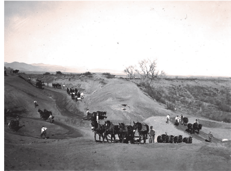
Exhibit 3-1: Photograph showing re-sloping of Canal. In 1933. Earth grading of the Canal using horse-and-slips, combined with manpower and simple tools, is reminiscent of the Canal's original 1879 to 1883 construction. Source: Denver Water, Album 41, p. 43, photo #3752.
