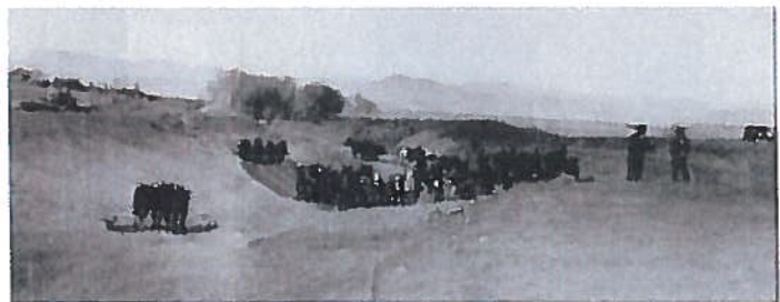
Historic photo of canal construction. Due to its relatively junior water right, the Canal never met the expectations of canal developers and farmers.
