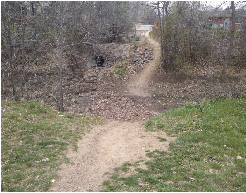
New Bridge at S. Franklin St.
