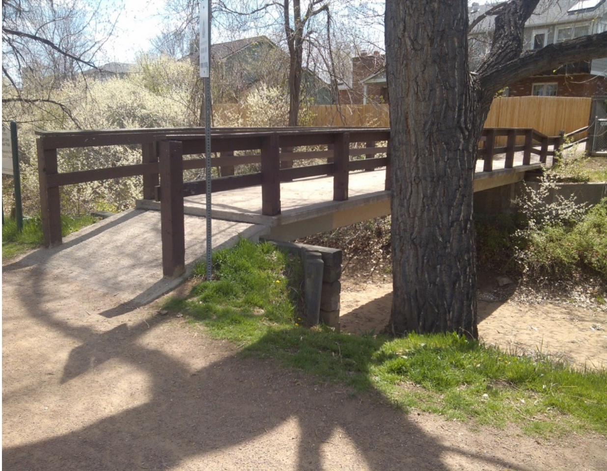
Bridge at S. Bannock St.
